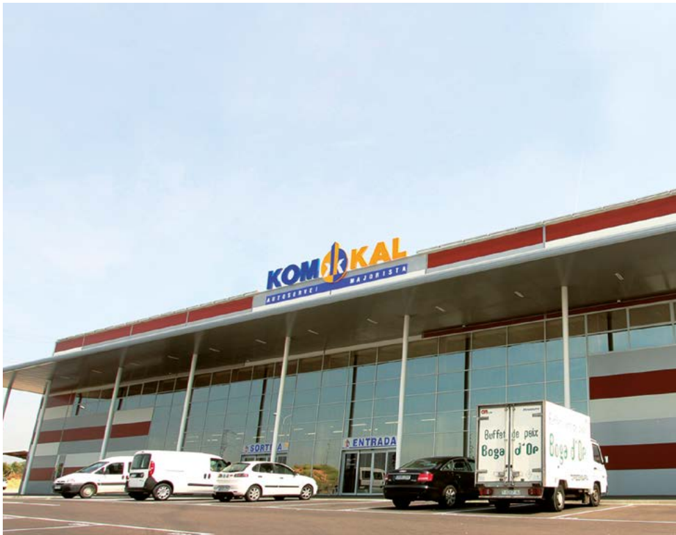
Komkal Industrial Building
